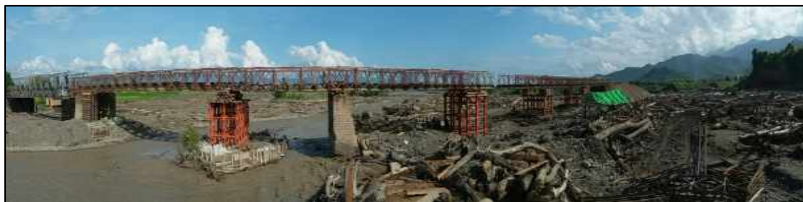
Repaired MyaungChaung bridge in Gangaw- Kalay road. Credit: Myanma Railway
